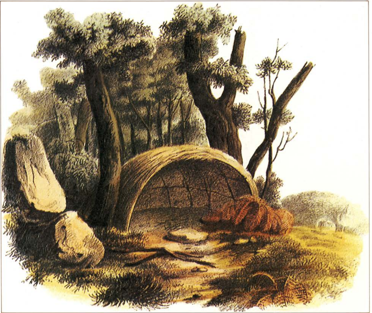
Nyungar hut drawn by de Sainson 1826. The family slept in a hut about 1m to 1.3m high and 2m across. Women constructed huts in less than half an hour, with flexible branches set in a semicircle, bent and tied with vines at the top, then support branches were woven or tied horizontally. Over the basketwork frame, paperbark or Xanthorrhoea leaves provided a roof. The opening and the hearth faced away from prevailing winds. D'Urville, Voyage de la corvette L'Astrolabe, Atlas historique.
